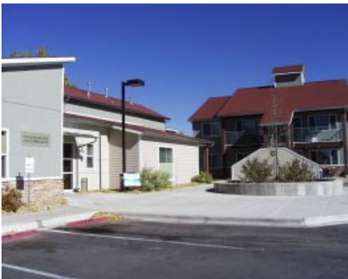
Plaza del Milagro is a 40-unit multi-family housing complex for migrant and seasonal farm workers in Greeley, Colorado. The complex has a childcare center and a community building on the 5-acre site, which is operated by Catholic Charities and Community Services of the Archdiocese of Denver.
