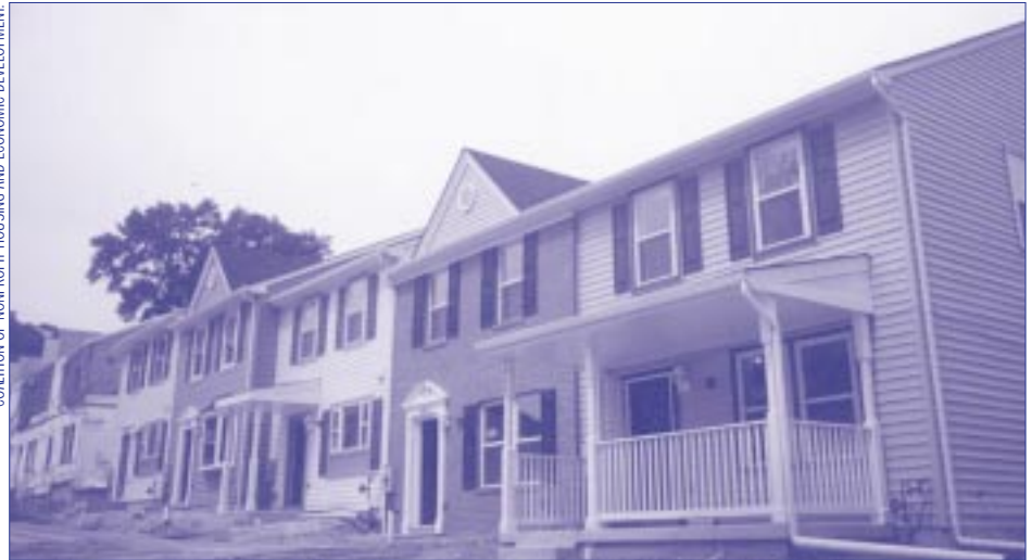
Chaplin Woods, D.C. This 22-unit new townhome community in southeast Washington, D.C. is located just two miles west of the Capitol. These homes were developed by Manna, Inc. and Marshall Heights Community Development Organization.
