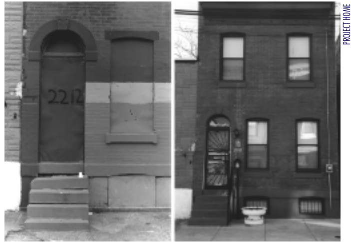
Rehabilitation of a vacant home in North Philadelphia is part of an 18-unit affordable homeownership initiative by Project H.O.M.E. Philadelphia has approximately 30,000 vacant buildings.
