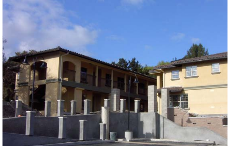
The Atascadero Senior Apartments are nearing completion and occupancy.
